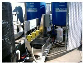
The ISD™ system enhanced groundwater with a nutrient-amended carbohydrate solution (CarBstrate™) prior to distributing it into the subsurface via two upgradient injection wells. Shallow groundwater was already anoxic due to the presence of Stoddard solvent, which had promoted partial dechlorination of PCE (as indicated by the presence of TCE, DCE, and VC prior to initiating the pilot demonstration). CarBstrate™ was selected as the electron donor due
